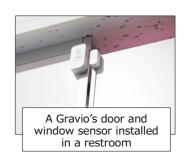
Kawasaki Frontale and Okaya Electronics adopted Gravio for the purpose of monitoring congestion and preventing the Three Cs. They developed the restroom usage visualization service, installing about 100 door and window sensors in the restrooms of Kawasaki Todoroki Stadium to enable visitors to monitor congestion with their smartphone and avoid crowding.
